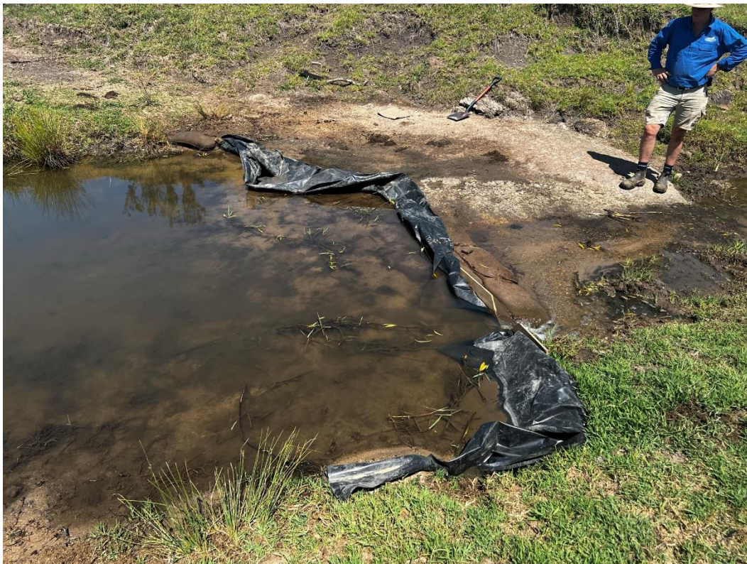
Figure 9 V-notch weir construction
